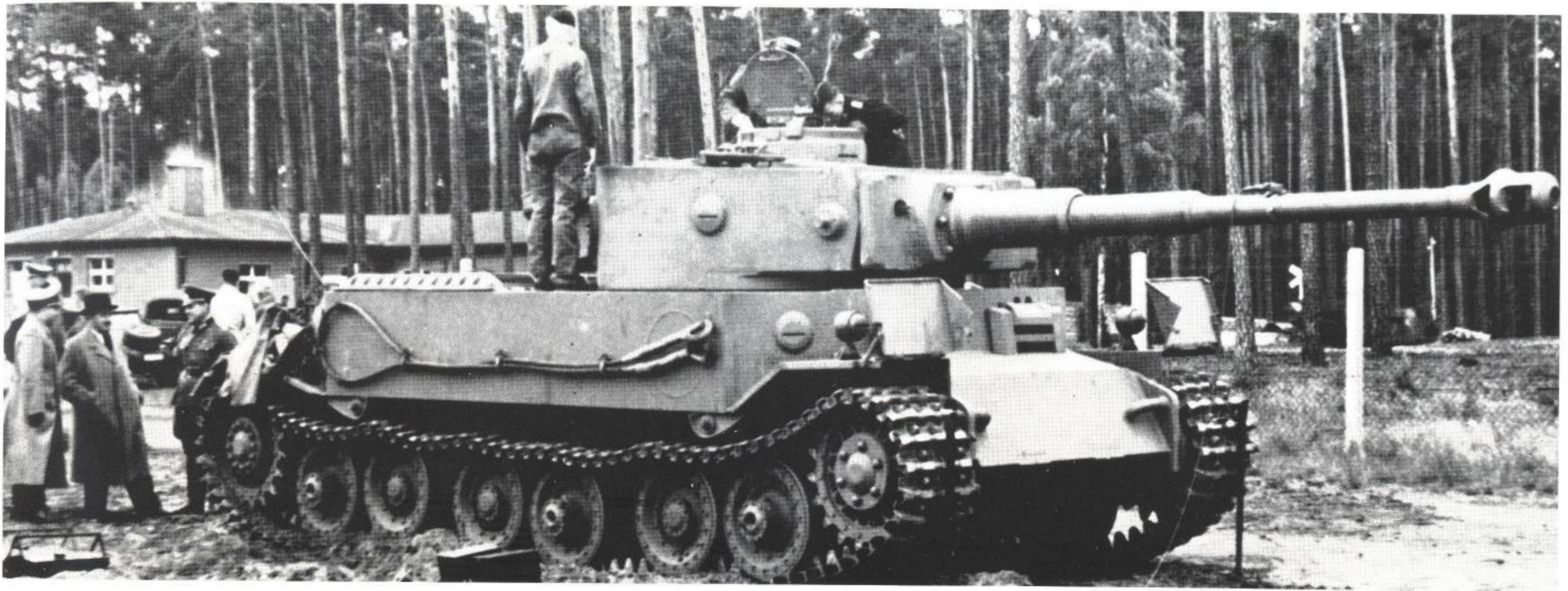
Above: One of the ten completed "Tiger P" tanks with the 8.8 cm L 56 KwK. At Hitler's order, the possible mounting of a heavier gun (10.5 or 15 cm) had also been discussed. At left in the photo is Prof. Porsche, in discussion with officers.
